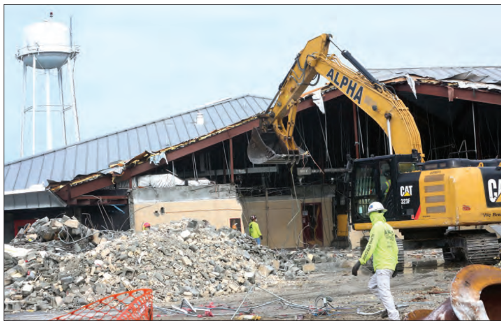
Demolition of the original Ahfachkee School took place in early March.
